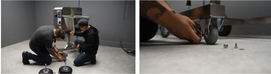
Unscrew the 4 bolts holding the caster to the underside of the bucket using a 7/16" socket or box end wrench
