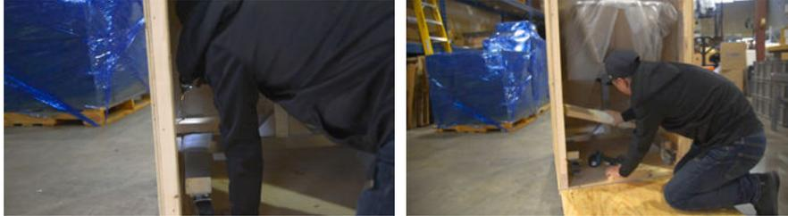
Unscrew and remove the 2x4 blocks holding the bucker in place inside the crate.
