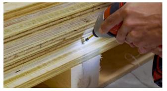
Locate and remove the screws that are securing the wooden blocks in place at each end of the machine.
