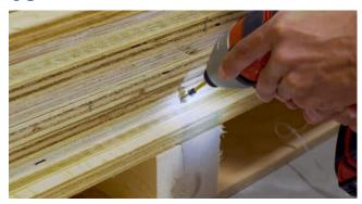
Locate and remove the screws that are securing the wooden blocks in place at each end of the machine.
